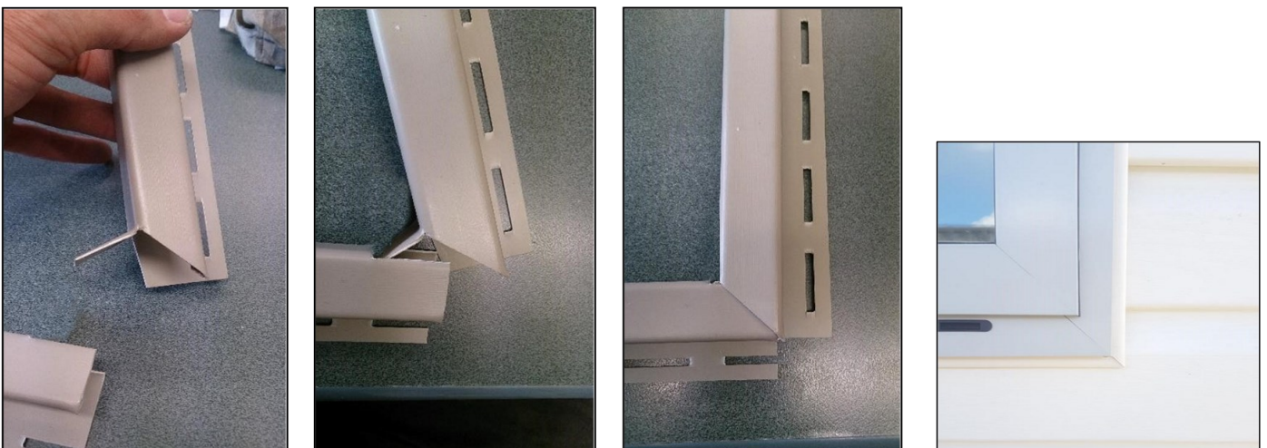
Diagram 1, cutting external corners for window sills
